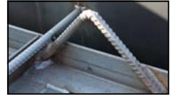
Transport hooks are welded in for ease of loading and unloading.
